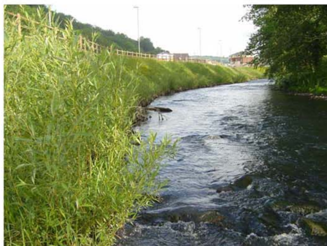
Above : Photo of the bioengineering works 1 year after completion
