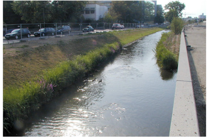
Development three months after installation. As the riparian plants mature they withstand higher floodwater flowing speeds or other impacts such as grazing or access by people.
