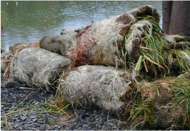
Plant carpets onsite ready for installation. The plants have developed a dens root system with runners and rhizomes.
