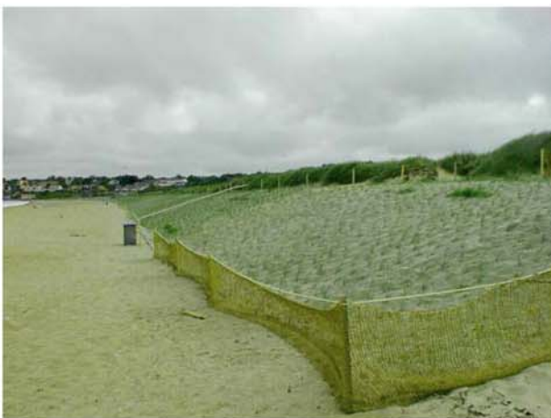
Vertical coir fence
