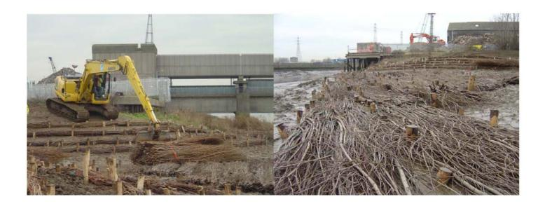
Photos: Brush packing Revetment Installation and (bottom right) 3 months growth
