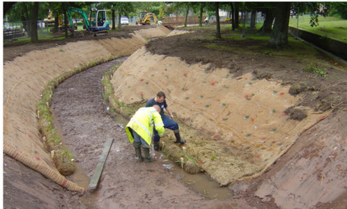
Above: Coir roll and NAG C125BN are installed
