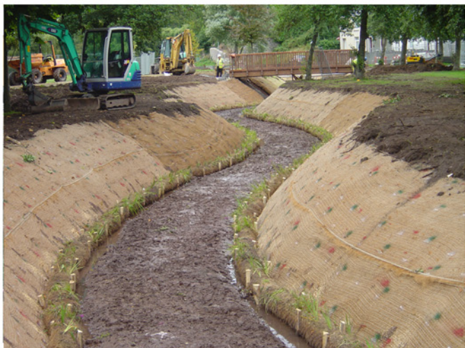
Below: Completed Bioengineering Works in the new cut channel
