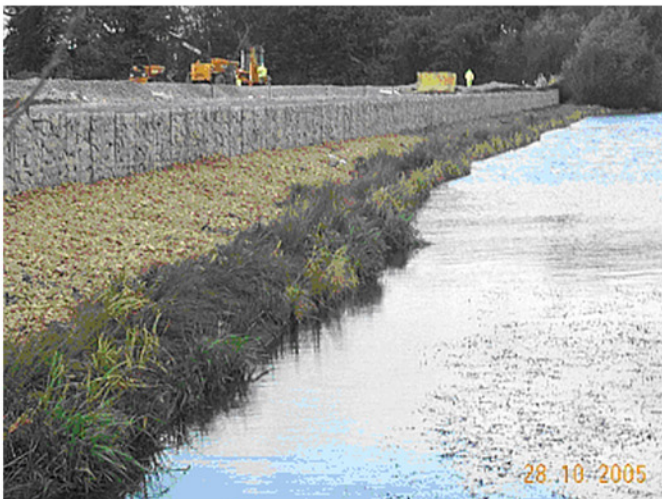
Above: The bioengineering materials after installation.
