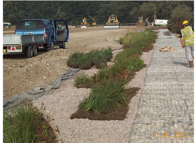
Above: The pre-established coir rolls and pallets are delivered
