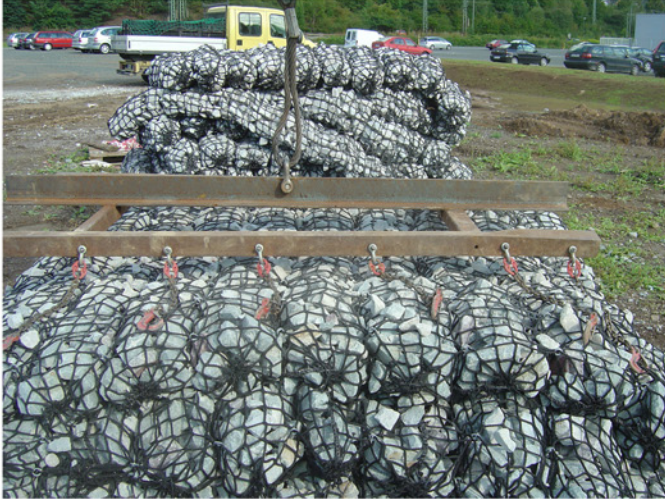
Delivery of the rock mattresses on the site.
