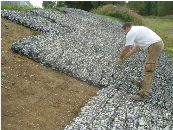
The single 2m x 2m – elements are interlocked with C – shaped clamps
